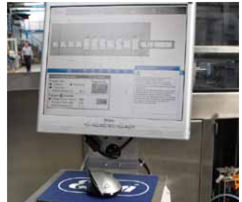
IPC control with operating screen
